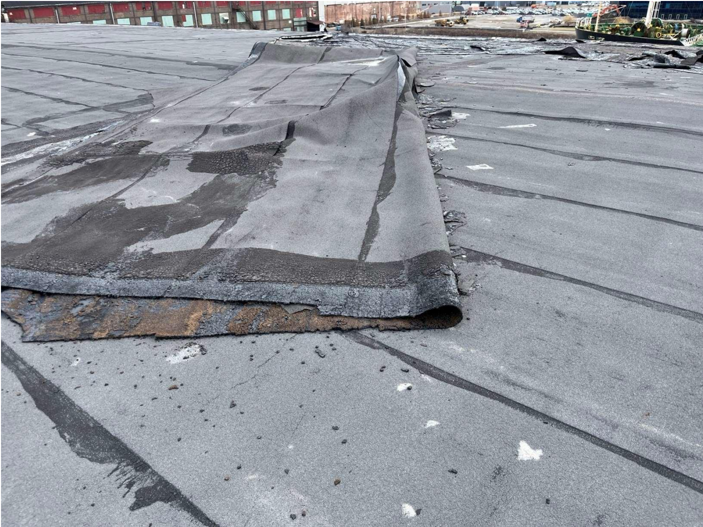
Y-2 Building Looking Southeast
