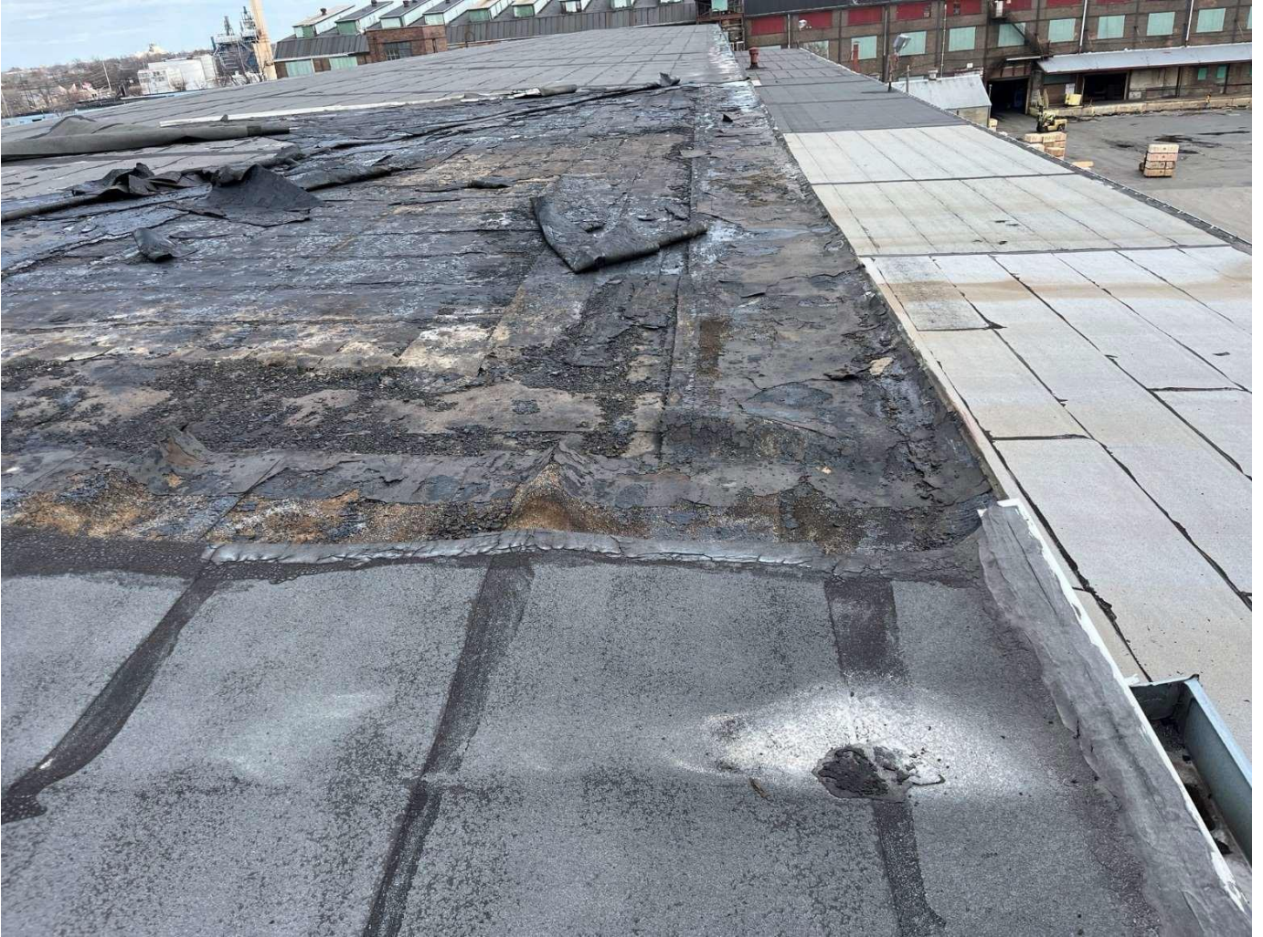
Y-2 Building Looking East
