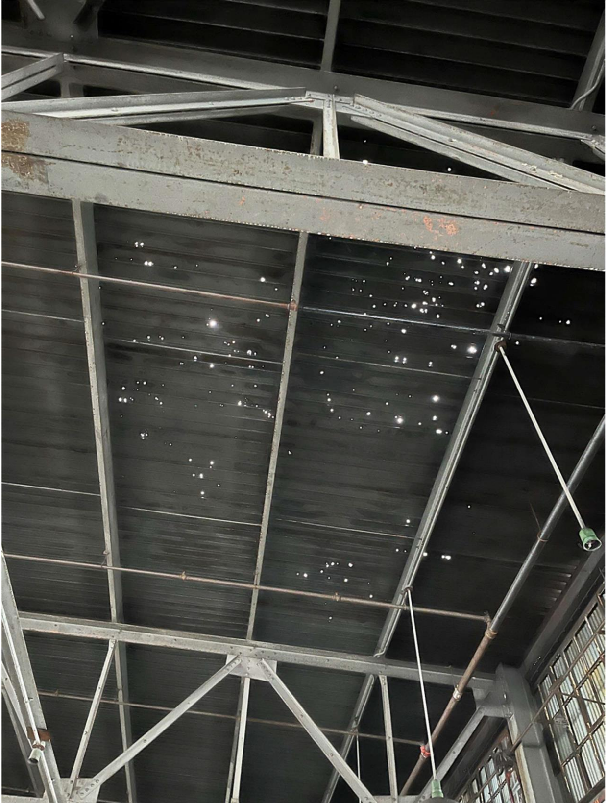
Y-2 Building Roof - Looking Up From Below
