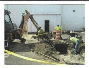
On Saturday, September 28, it was reported to us that the 8" pipe had failed catastrophically that morning. The tenant had to shut down all fire water to Pier 5 and put the entire facility on a fire watch. Our maintenance staff responded and were successful in closing a valve to isolate the leak to just Warehouses 2 and 3. We then hired the low bidder to perform an emergency repair which was completed on October 2nd, 2024.
