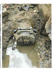
When the water was turned back on, a second leak appeared in a different location under the floor inside Warehouse 2. An emergency repair was then performed to that 8-inch line in order to isolate it and abandon it below the floor. That work was completed on October 10, 2024, and enabled Warehouse 2 to be returned to service.
