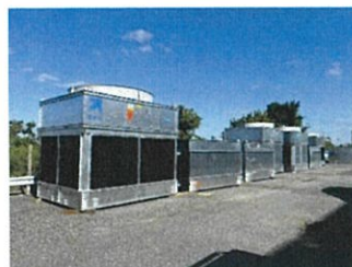
New Rooftop Equipment Delivered On-Site
