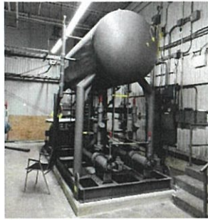
Chilling Plant – New Equipment Installed
