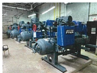
Chilling Plant – New Equipment Installed
