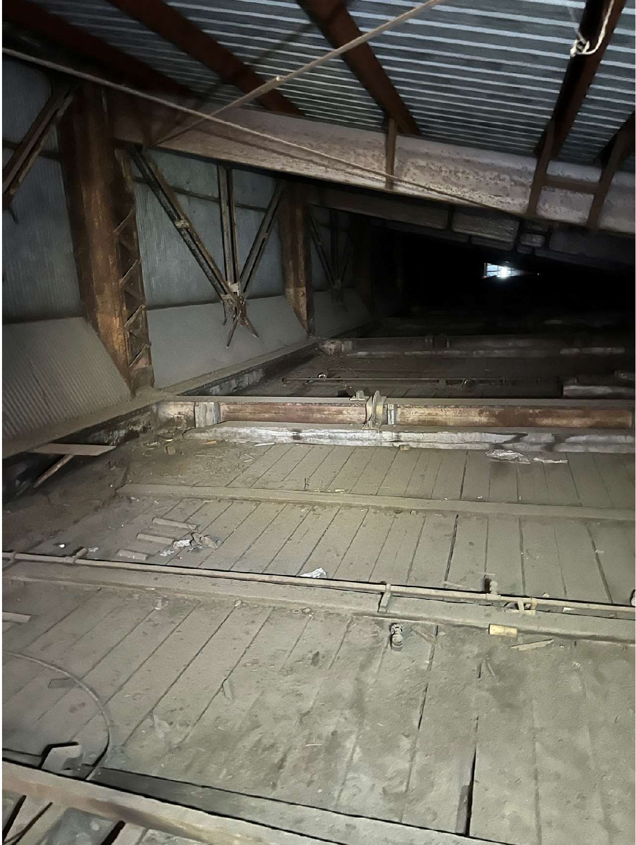
Photo No. 1 – Attic Space above West Gallery – Looking South
