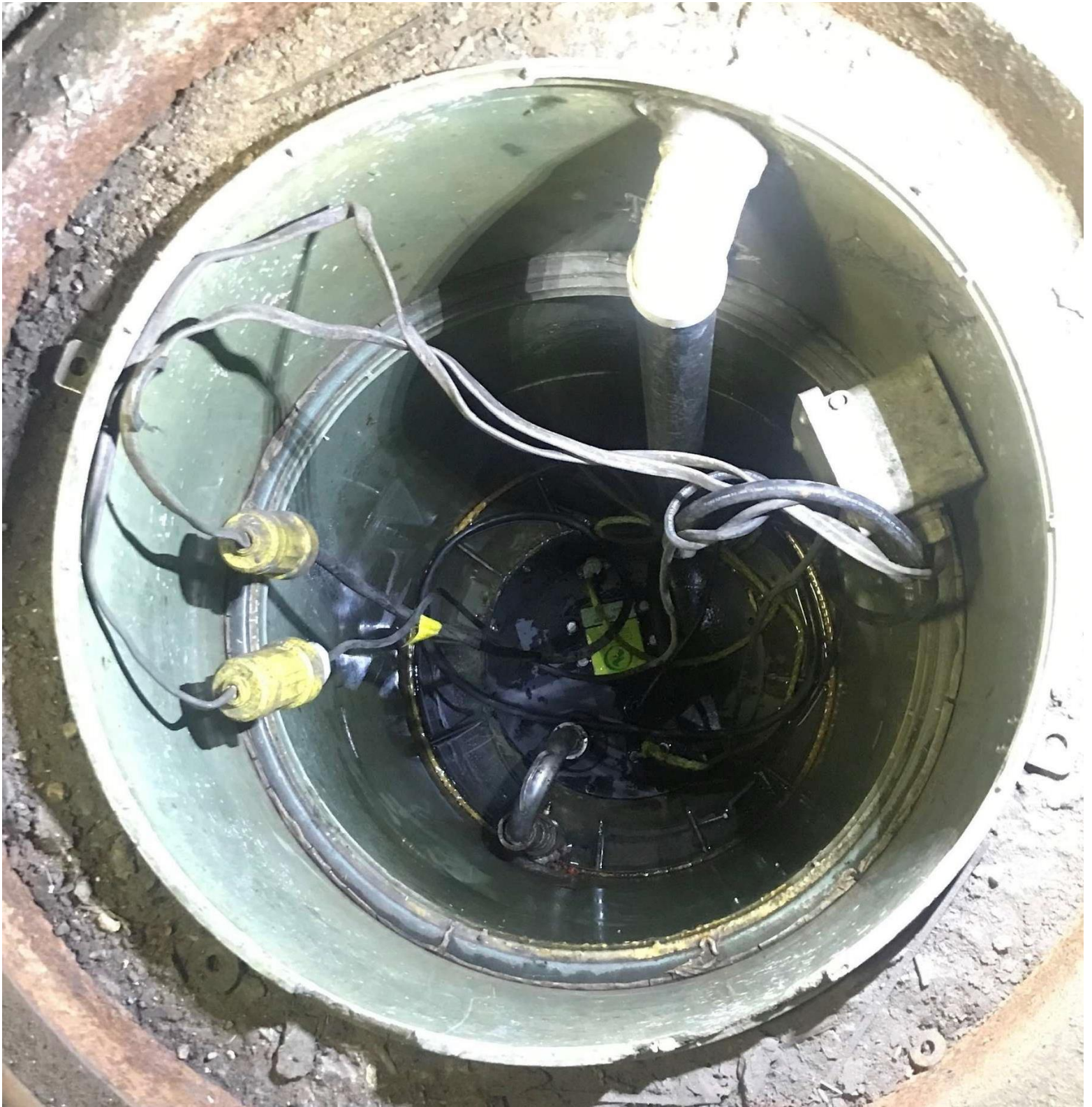
Existing "Canned" Pumping Station Wet Well
