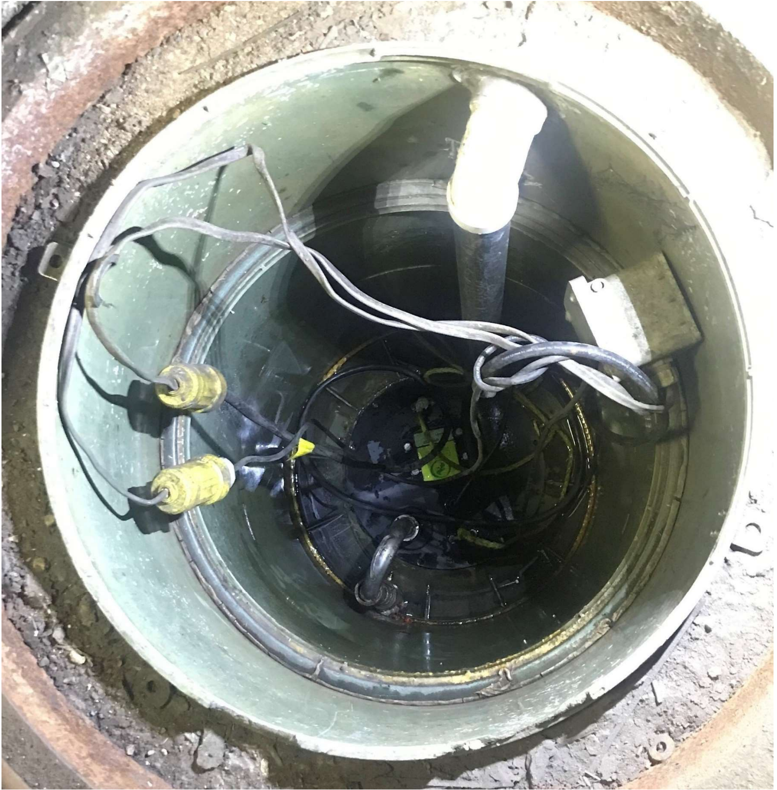
Existing "Canned" Pumping Station Wet Well
