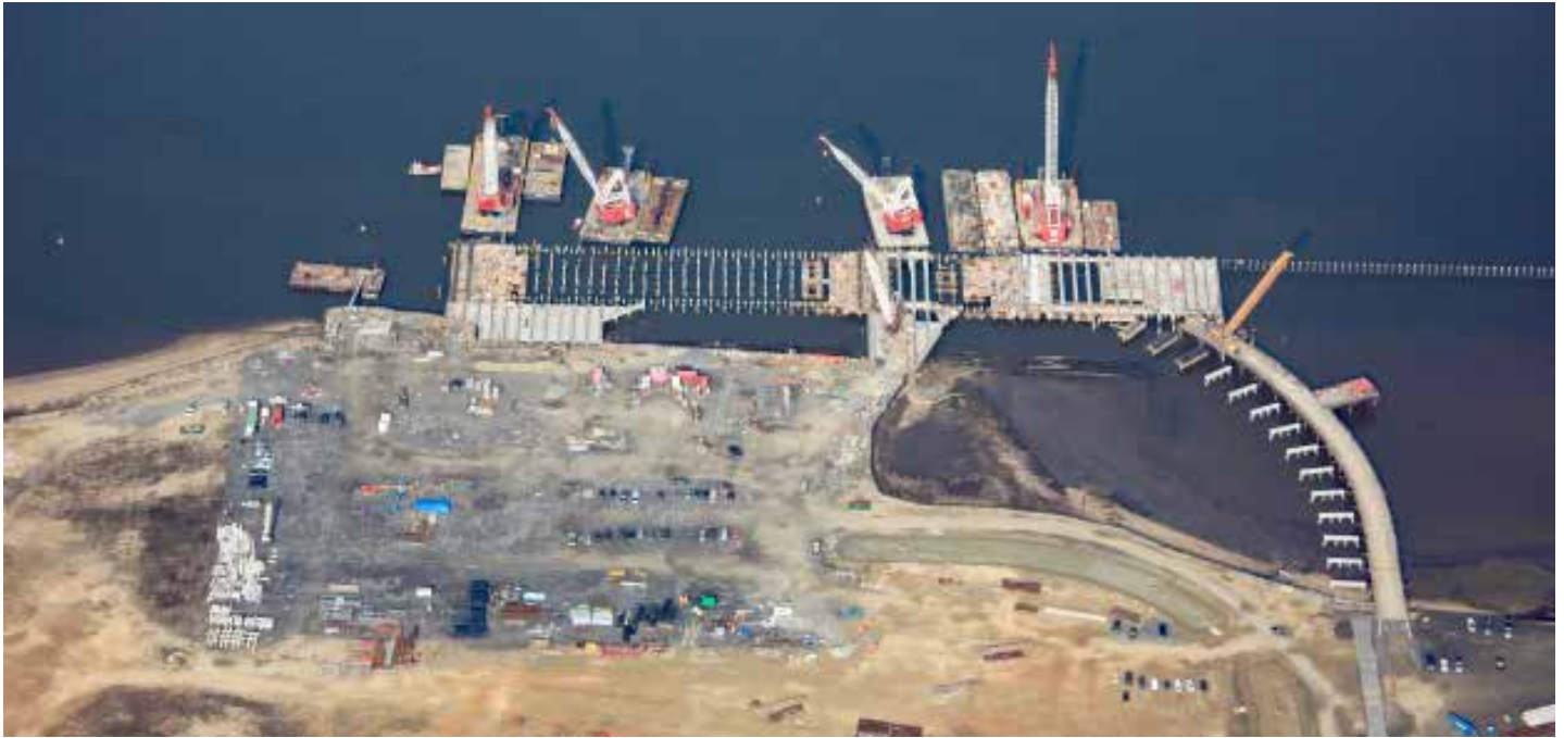
The wharf at Paulsboro Marine Terminal nears completion in the fall of 2016.
