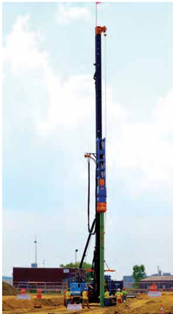
Pile driving one of the 4,000 pilings at Broadway
