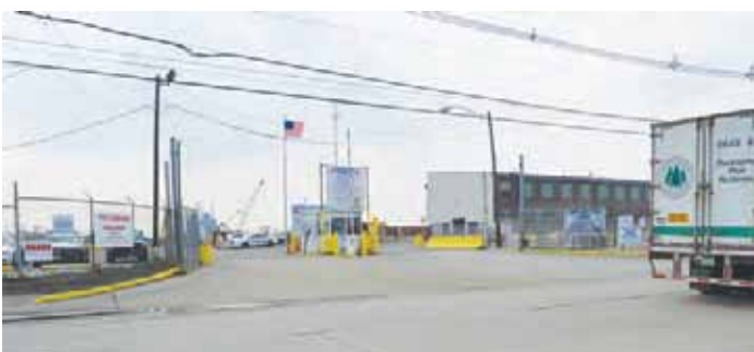
Above: Holtec's Dr. Kris Singh and NJ Lt. Gov. Kim Guadagno greet Camden Mayor Dana Redd and other guests at the ground-breaking ceremony. Below: Holtec's construction gate at Broadway
